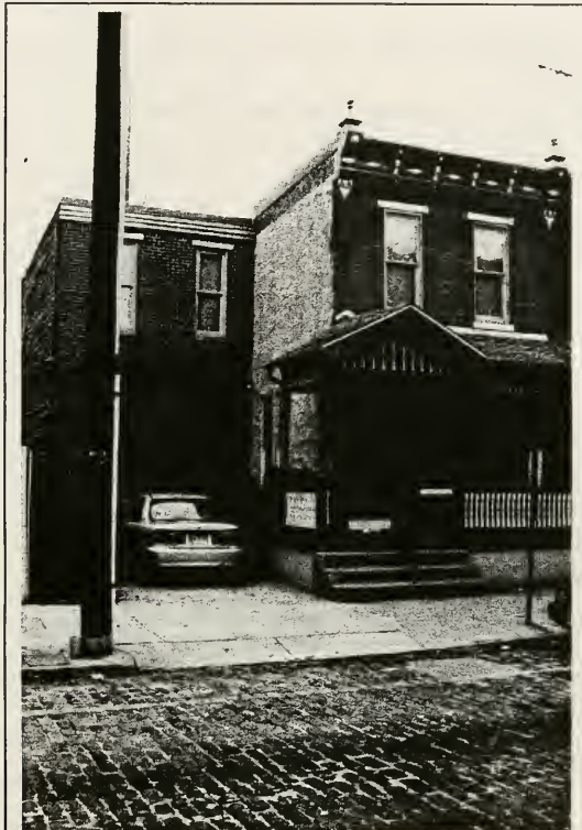
Figure 14. 409 South 7 th Street. Front elevation showing the side addition.
